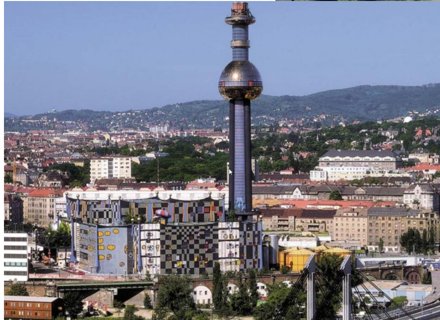
Spittelau waste treatment station, Vienna, Austria
